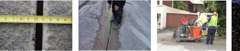
Deep: 70 to 300 mm Width: 10 a 30 mm Trench opened with specilized equipments that has cut disks Fill the trench with quick drying grout
